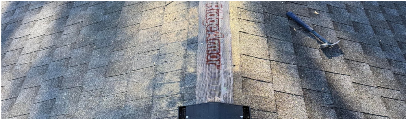
Actual RidgeArmor field installation. RidgeArmor protects the structural ridge slot before the separate compatible continuous ridge vent and cap are installed.
