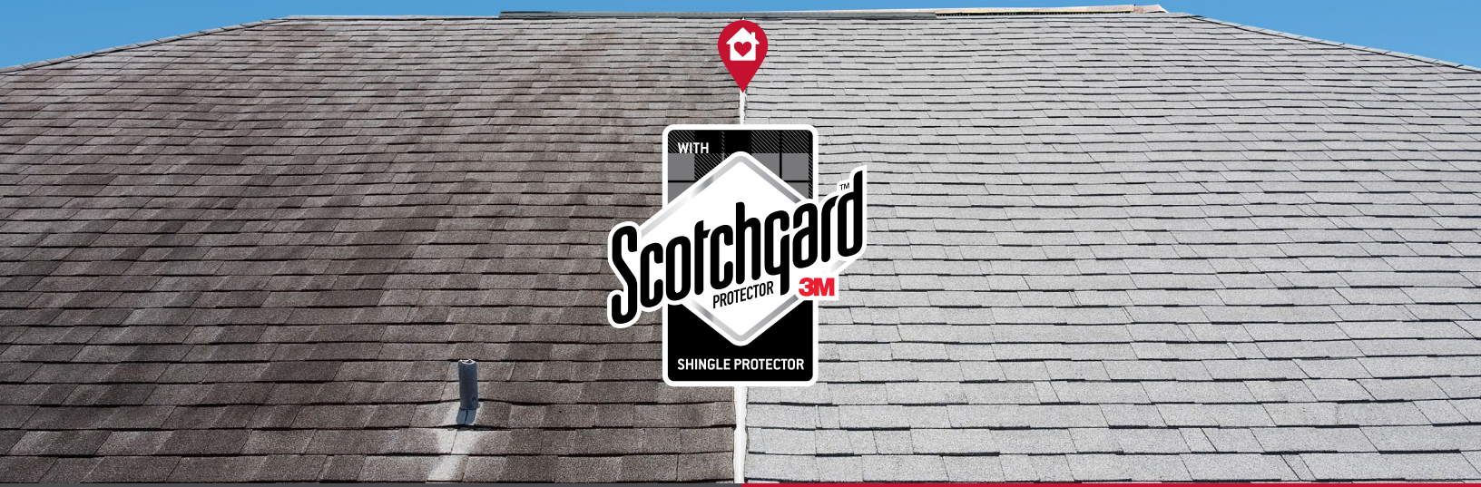
SHINGLES WITH BLACK STREAKS CAUSED BY ALGAE
