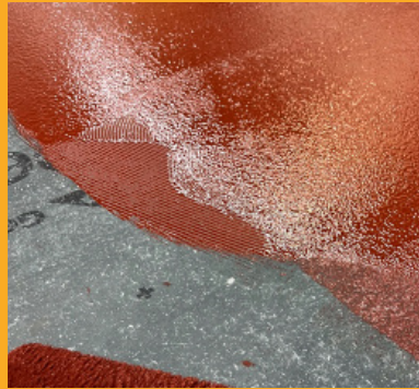
BACK ROLLED WITH 3/8" PRESATURATED NAP ROLLER
