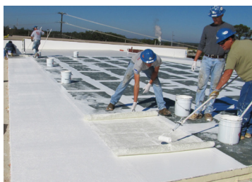
Step 5 – MEMBRANE APPLICATION
