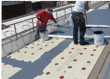
Step 5 – MEMBRANE APPLICATION
