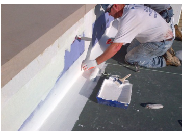
Step 4 – DETAILING/FLASHING
