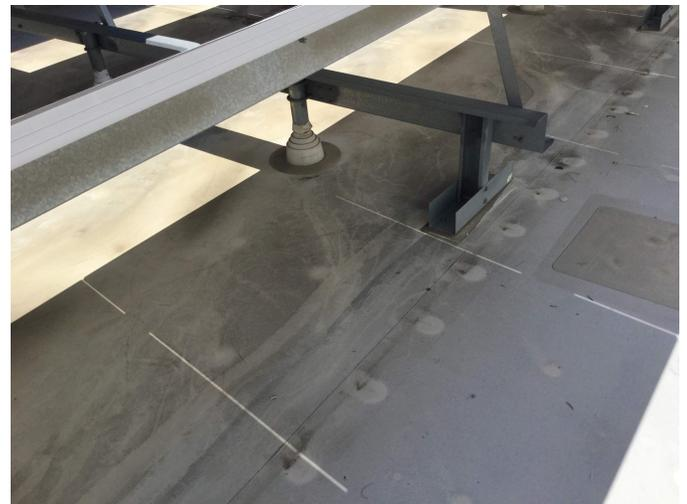
Examples of damage to a TPO roof from solar arrays.
