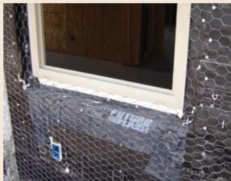
*FutureFlash® is ideal to effectively flash complex recessed window assemblies to prevent water damage.*
