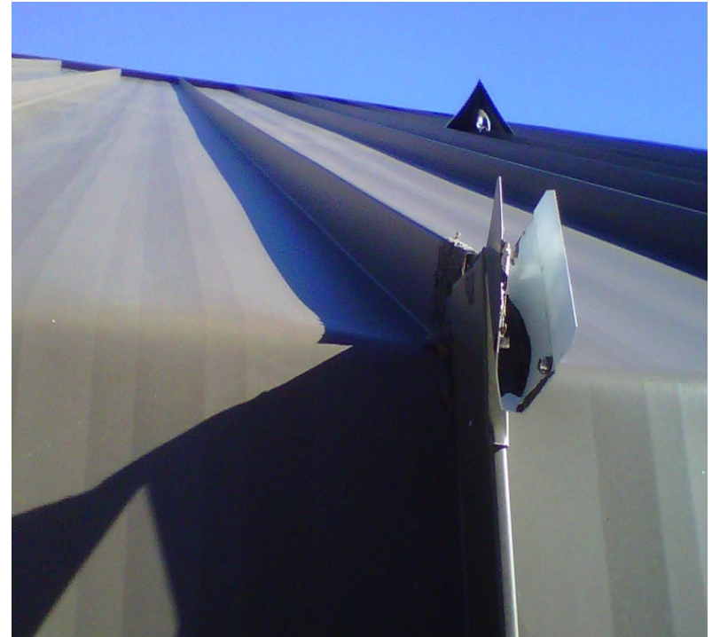
Image of failed knee joint in snow country.
