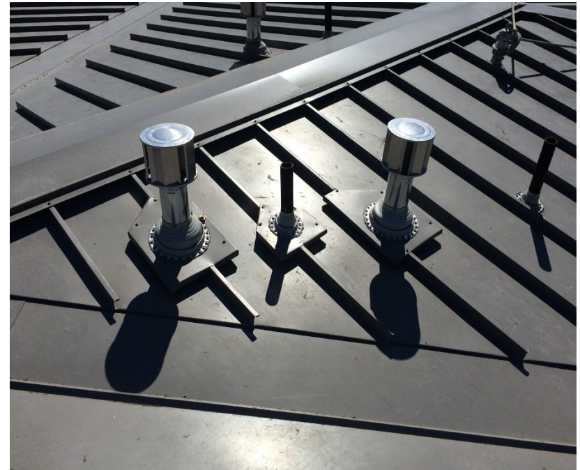
Correct: Cut Rib Detail
