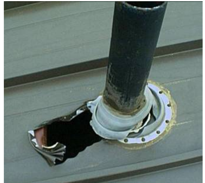
Drag load on pipe penetration. Pipe needs to be secure from underneath.
