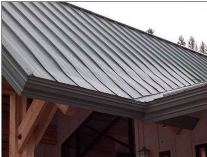
Ribs crushed due to inadequate valley width.
