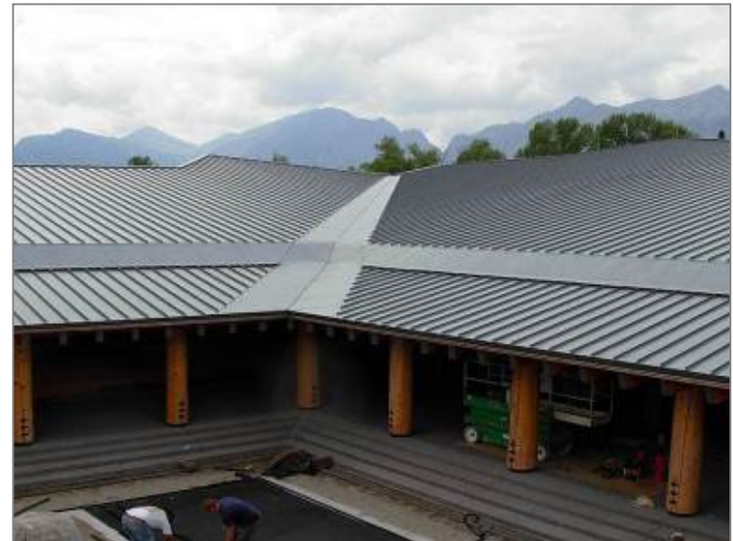
Snow conditions require special valley design.
