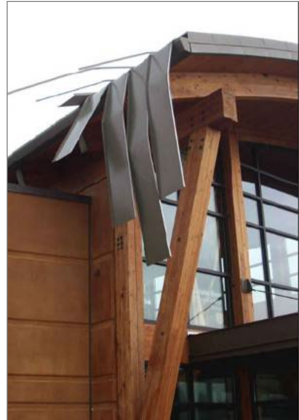
Damaged panels caused by snow drag load.
