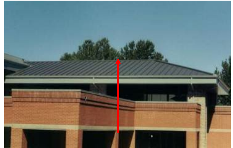
Dark Color - Cool Roof Heat is reflected into the atmosphere rather than into the building
