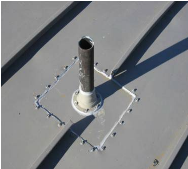
Incorrect: Standing Seam Penetrated
