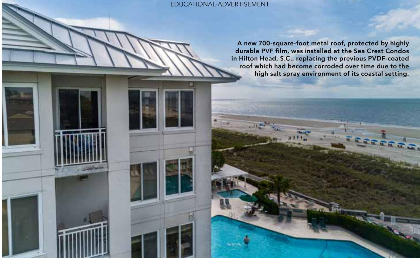
A new 700-square-foot metal roof, protected by highly durable PVF film, was installed at the Sea Crest Condos in Hilton Head, S.C., replacing the previous PVDF-coated roof which had become corroded over time due to the high salt spray environment of its coastal setting.
