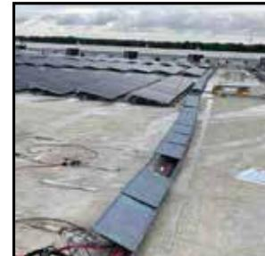
Proper design and installation of PV systems are critical. Above is an EPDM ballasted roof that has compromised wind uplift performance due to reduced ballast to accommodate structural limitations and a ballasted PV array that failed due to insufficient wind uplift resistance.
