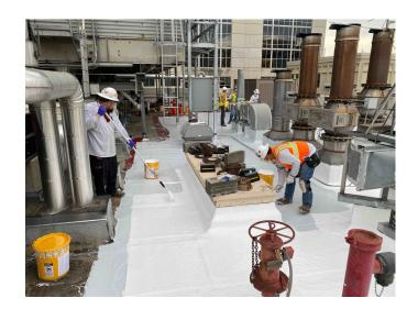
An existing roof can be significantly enhanced by a new Sikalastic® RoofCoat system. New recovers can prolong the life of:
