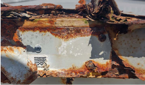
Coated roof edges prior to replacement
