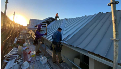
During Tedlar® roofing installation
