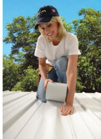
*Peel & Seal® is an ideal choice as a flashing material around chimneys, roof vents, stack pipes and other difficult to waterproof items. Peel & Seal® can also be used to completely cover, flash seams or repair metal roofing systems.*
