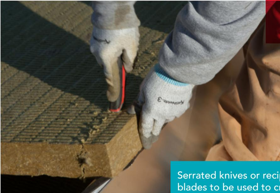
Serrated knives or reciprocating "serrated" blades to be used to create cleaner cuts and reduce waste and dust on the jobsite.
