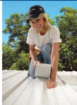
Peel & Seal® is an ideal choice as a flashing material around chimneys, roof vents, stack pipes and other difficult to waterproof areas.
