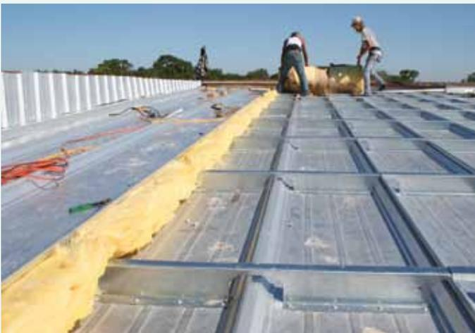
A trapezoidal standing seam roof being installed over trapezoidal standing seam roof with optional insulation.
