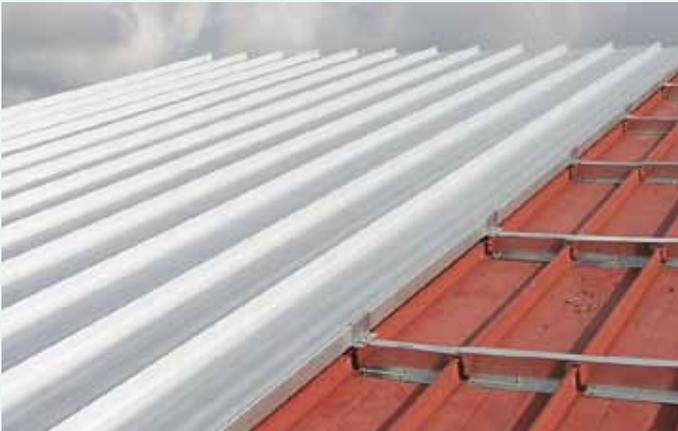
Vertical rib standing seam roof being installed over an old vertical standing seam roof.
