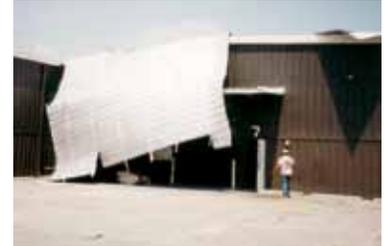
Actual resulting failure showing "peeled" roof.
