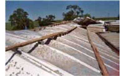
Failure of 2 x 4's on a wood framed roof.
