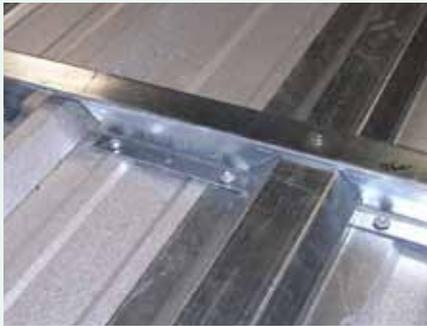
When Roof Huggers are attached to Sub-Rafters (See page 7) they are usually attached with  $\frac{1}{4}$ -14 drill tip 3, 1- $\frac{1}{4}$ " long. Denoted  $\frac{1}{4}$ -14 x 1- $\frac{1}{4}$ " Tek-3. The number of fasteners varies.
