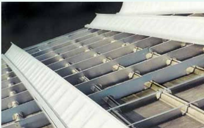
*Use 2 sizes of ROOF HUGGERS to remove a step in an old roof.*
