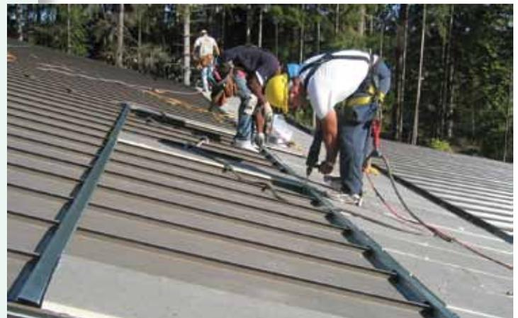
***Roof Huggers being installed with rigid insulation.***
