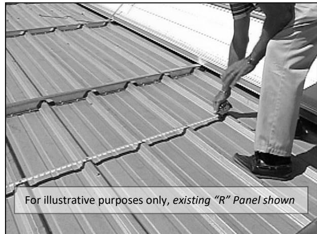
In order to assist you in the process, Roof Hugger has a specially designed cardboard "Template" that will help identify if the roof is one of the four most standard profiles shown above. You can obtain a template at no charge from Roof Hugger, Inc. by calling 1-800-771-1711.
