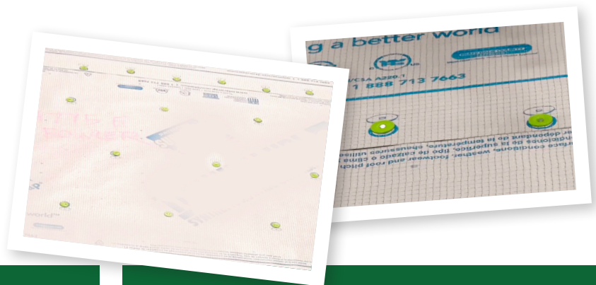
6" overlap at laps with 6" o.c., staggered
