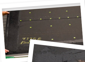
Lay starter strip into roof cement (1/4" over edge)
