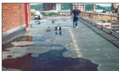
New York Housing Facility 40,000 sq.ft. EPDM (Rubber)
