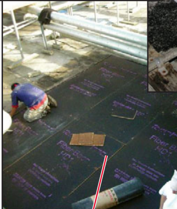
Proper cleaning to each substrate spec
