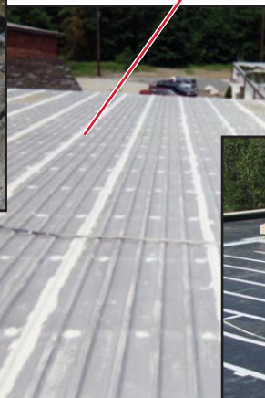
Completely re-flash and seal all seams on all substrates
