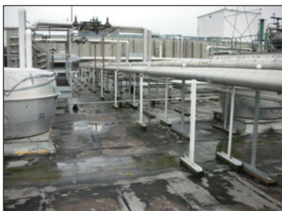
Missouri Food Processing Facility 112,000 sq.ft. Modified Asphalt
