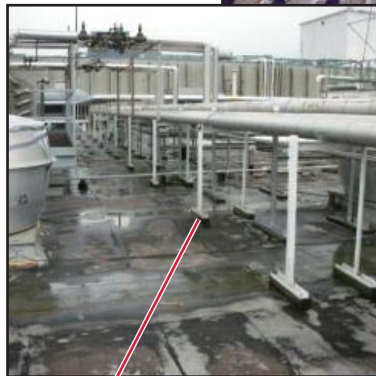
Multiple penetrations – ideal for fluid-applied roofing
