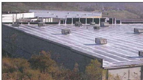
West Virginia Retail Facility 40,000 sq.ft. EPDM (Rubber)
