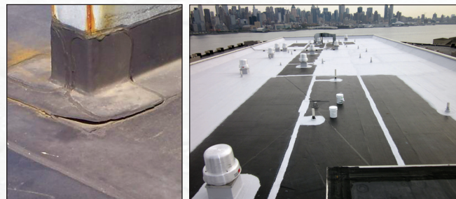
Seal all seams, splits and penetrations
