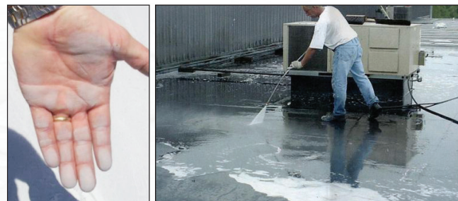
Clean surface and neutralize chalking
