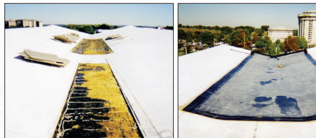
Repair substrate integrity as necessary
