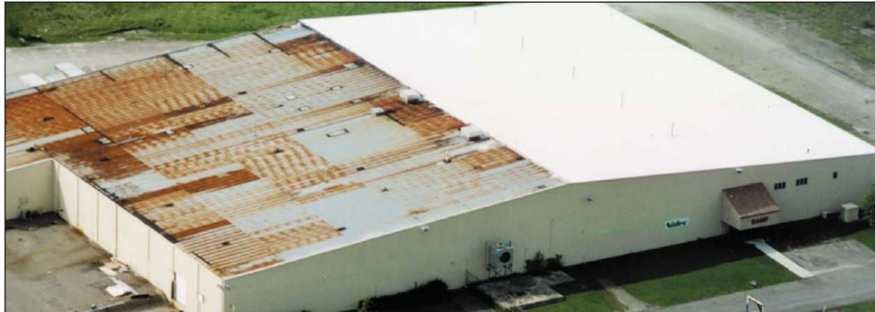
Leaky, rusting metal substrates are converted to seamless, sustainable cool roofs.
