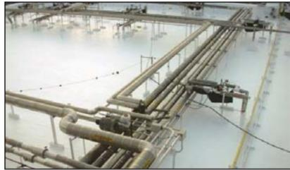
This asphalt roof with multiple supports and penetrations was a costly nightmare for traditional roof replacement, but was efficiently reroofed with a seamless, fluid-applied ASTEC® Re-Ply™ System.
