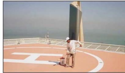
This concrete roof with a helicopter pad in Kuwait City was cracking in the hot, salt mist climate. ASTEC® Re-Ply™ fluid-applied roofing bonded directly to the restored concrete, producing a single, stable and sustainable new surface.
