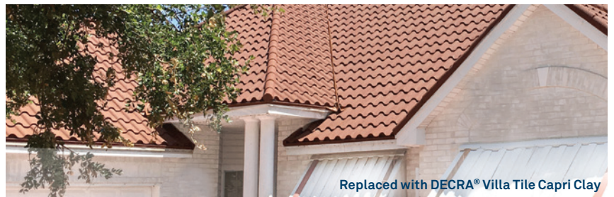
Clay tiles struck by hail.
