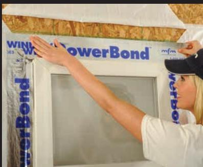
WindowWrap® PowerBond is composed of a silver polymer film that is coated with an aggressive PowerBond Broad Spectrum Adhesive. This advanced system bonds to all common building and window materials – even at 25°F.
