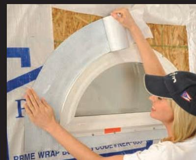
The unique design of WindowWrap® Flex PowerBond is the ideal solution for sills, arched windows, doors and irregular shapes. This product is impermeable to water vapor, moisture, insects and air.
